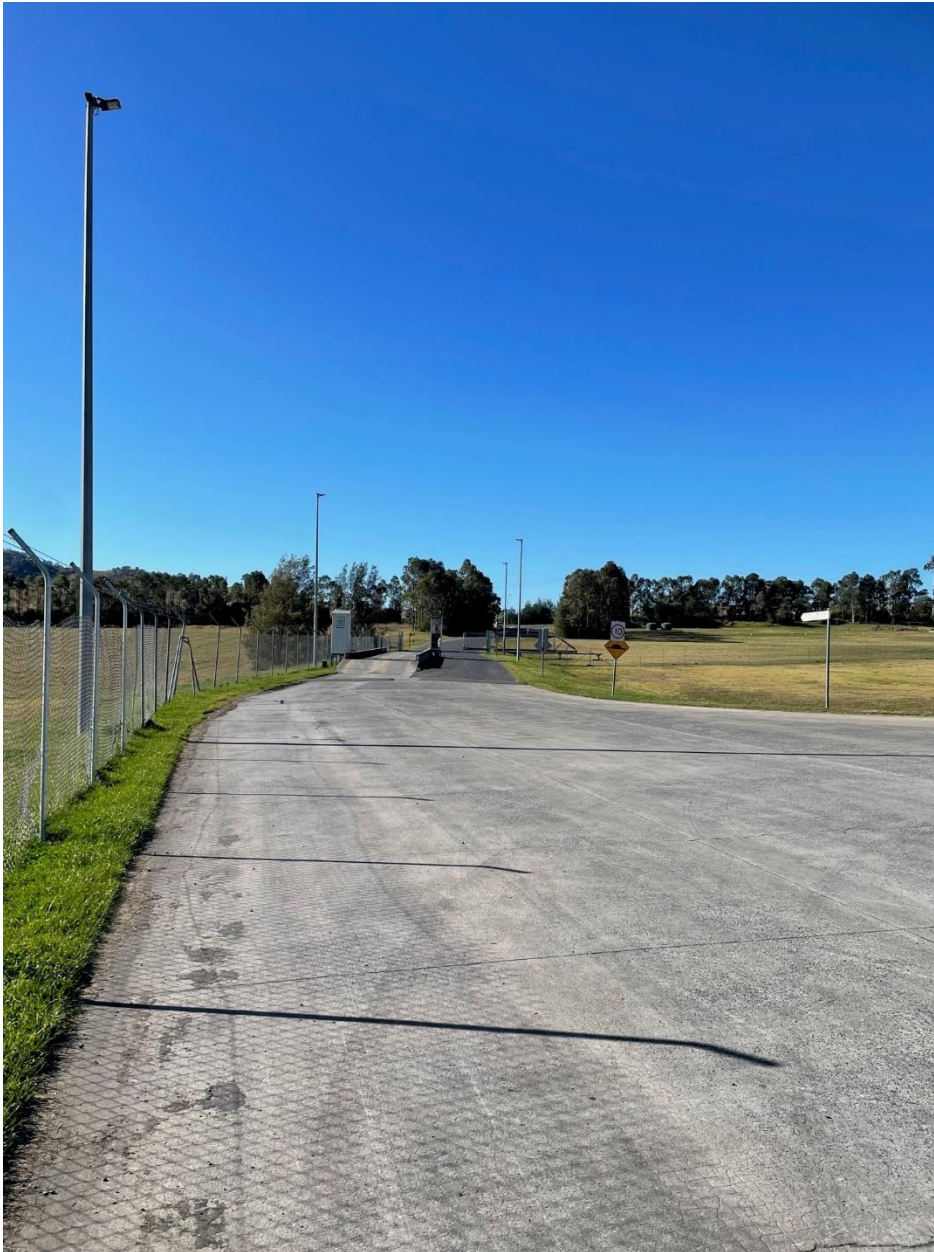
Photo 3 Weighbridge and Site Entrance
